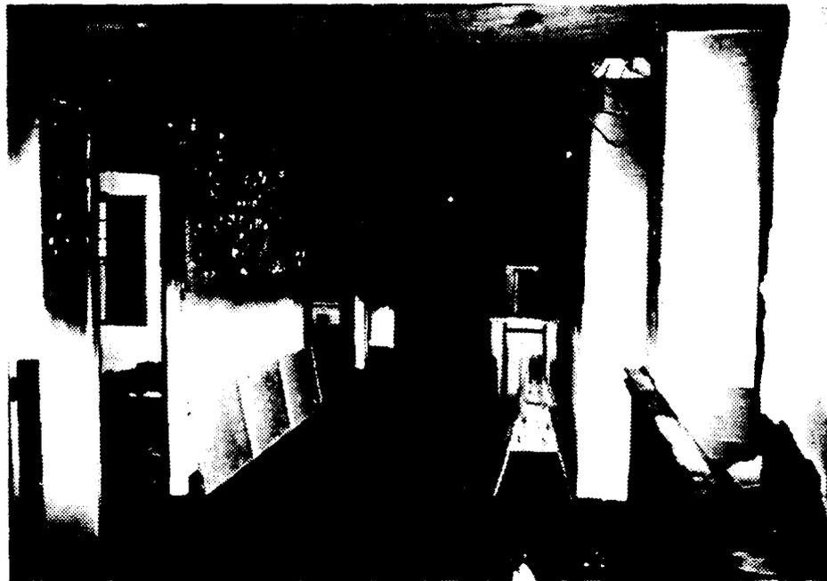
Figure 10. View from the the front desk into the corridor towards the room of origin. Note the descending smoke mark level on wall towards the area of origin.
