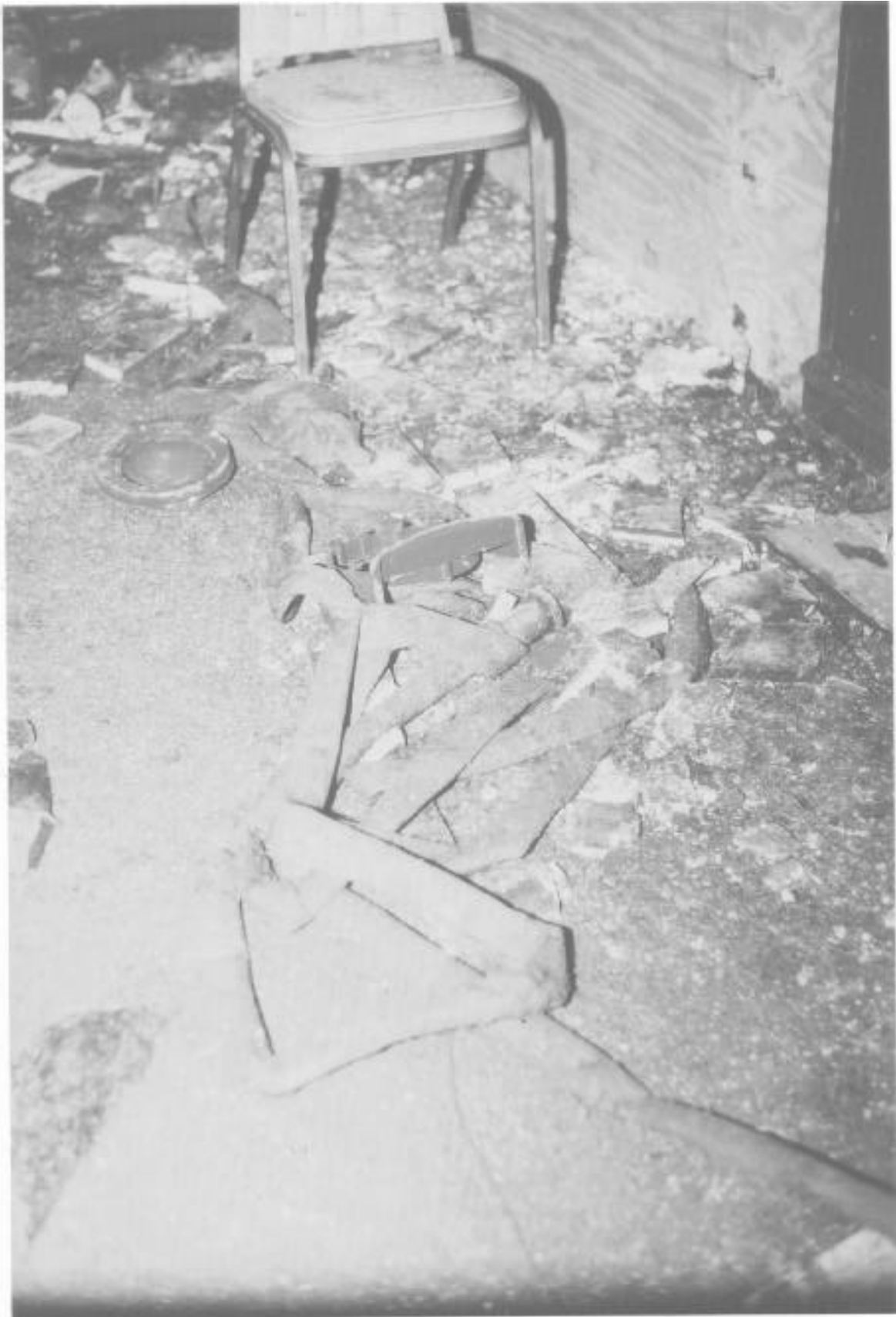
Remnants of occupant use standpipe hoseline used by Engine 7 and Truck 13 firefighters in the initial attack. Note the plastic adjustable-stream fog-nozzle attached to the end (near center of photo).
