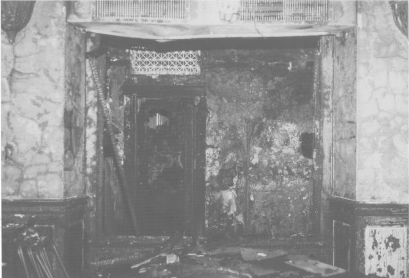
Entrance to ladies room adjacent to the dutch-style service door to the bar (room of fire origin). Note the air return register over the door and the air supply register over the opening to the dining room.
