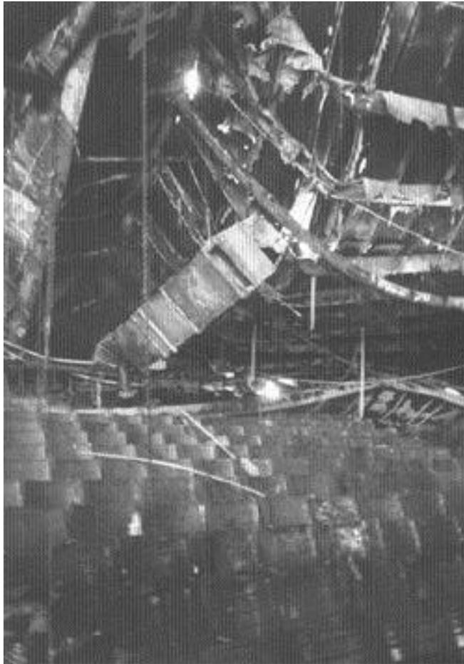
**This picture was shot from the direction of the stage showing the roof and structural steel failure in the auditorium. The heat level is indicated by the damage to the seating**
