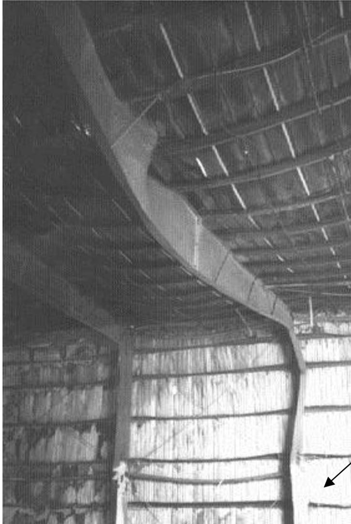
Visible here is buckled steel from the wall and roof of the prop maintenance building. The heat traveled horizontally from the stage roof through the 40-foot hallway to the building.
