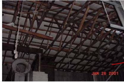
WOODEN TRUSS ROOF THIS ROOM ONLY!
