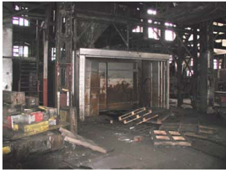
MACHINERY / HOPPER (RED SECOND STORY STRUCTURE)
