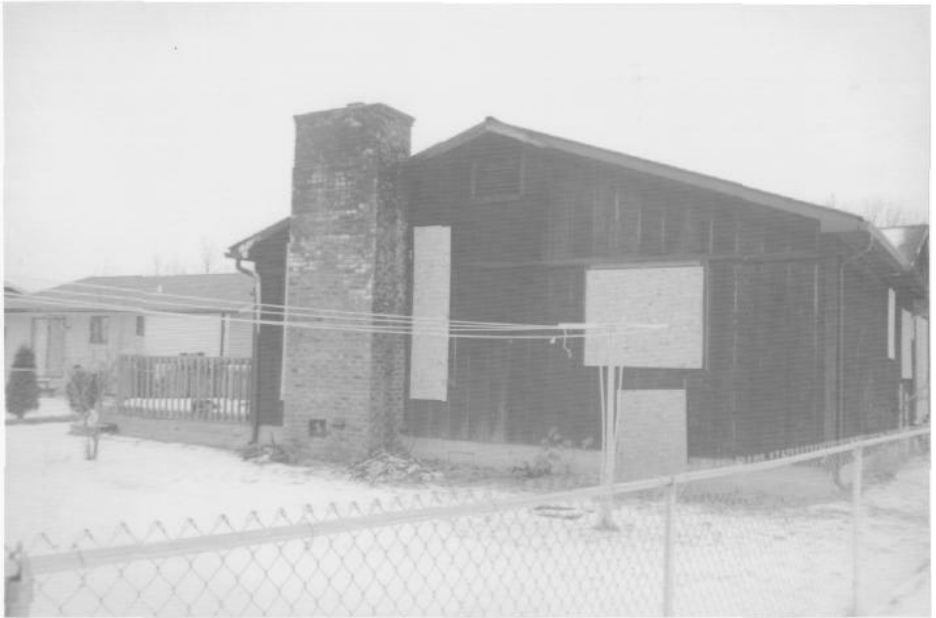
Rear view of the home, with no evidence of fire venting through the rear bedroom window.
